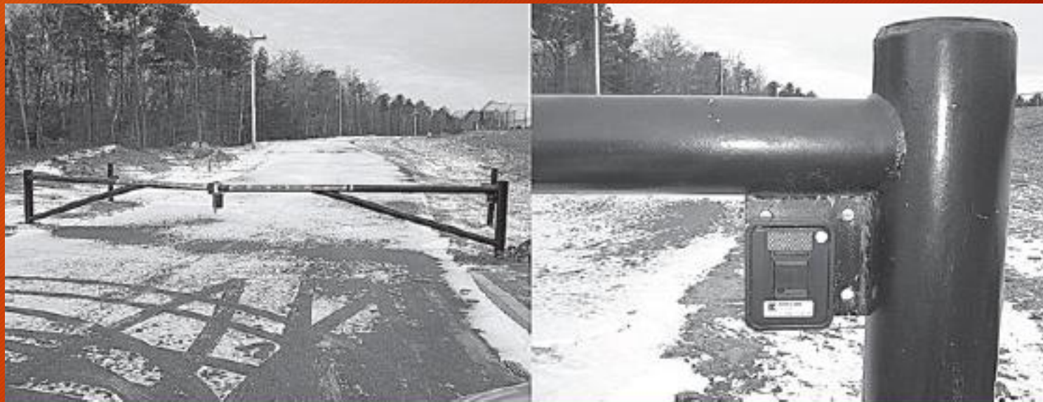
Example of gate access and access box.
